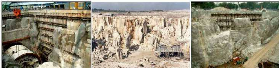
Underground Hazards in KL Limestone - Varying rock head conditions and sinkholes formation
