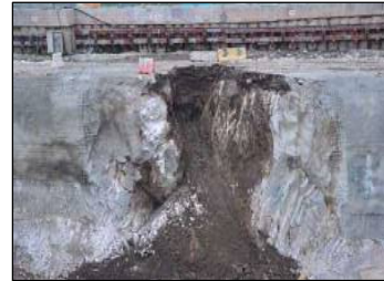
Cochrane Station Shaft KVMRT 2012
