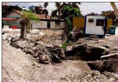
Underground Hazards in KL Limestone - Varying rock head conditions and sinkholes formation
