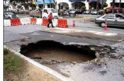
Underground Hazards in KL Limestone - Varying rock head conditions and sinkholes formation
